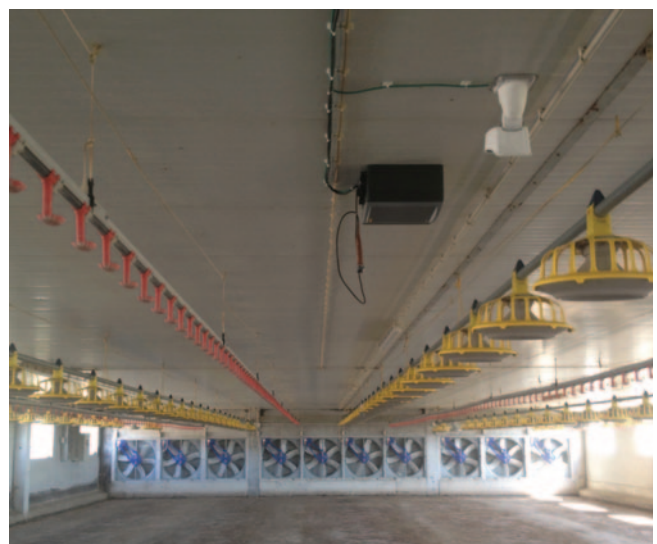
Sound monitor and camera system installed in a broiler house
